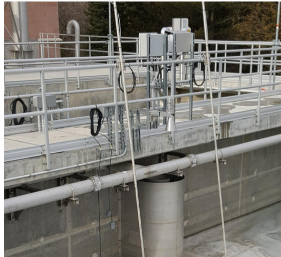
Figure 2: Pipes, tank walls and other obstructions around the sensors mounting.
