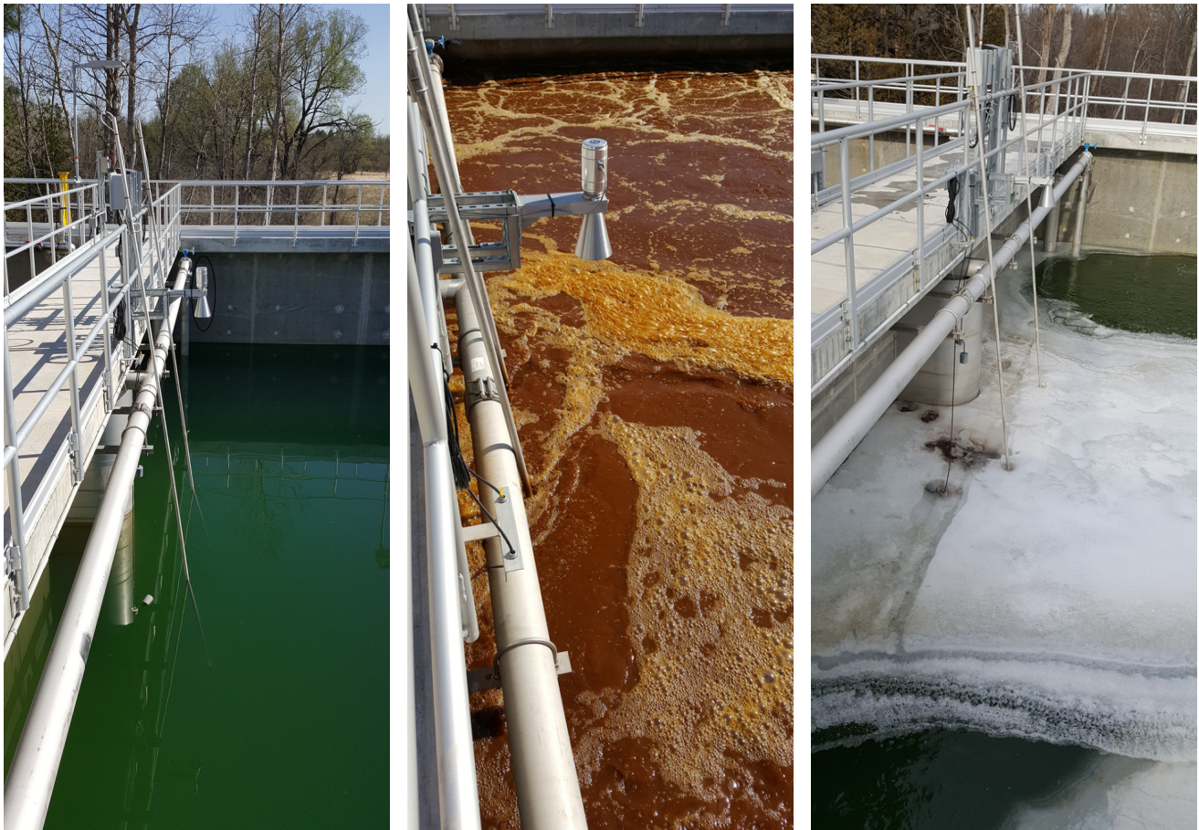
Figure 4: ABM radar level sensors installed in SBR basins measuring through foam and ice.
