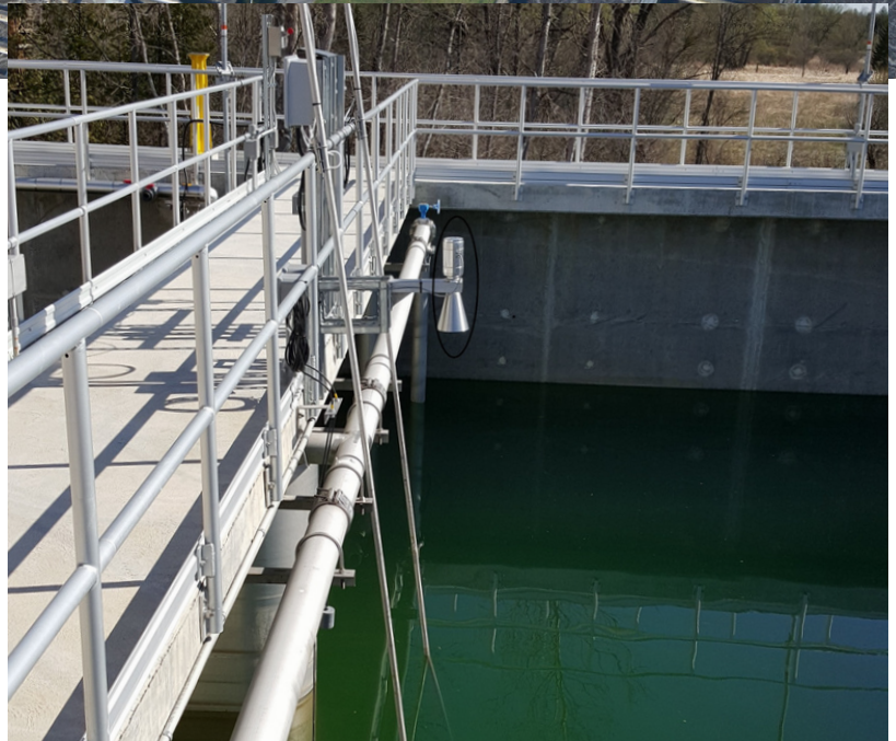
Figure 1: ABM's Non-Contact Radar Level Sensor installed in the SBR basin.
